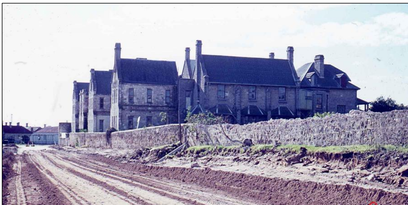
1968 Ord Street under construction
