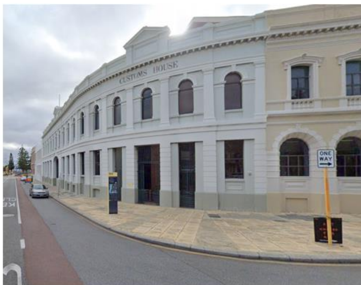
Former Falk Building 2024
