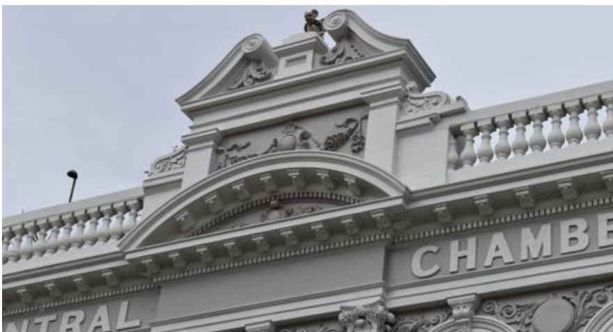
Detail of the Central Chamber's building
