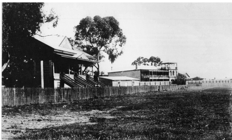
HISTORIC PHOTOGRAPH OF GILBERT FRASER RESERVE – The picture shows the wooden picket fence built inside the ground. The Gresham Hotel is in the right of the photograph, with the press box between it and the grandstand. The entire oval was originally enclosed by an eight-foot picket fence and the playing arena by a three-foot picket fence. The outer fence was replaced by cyclone wire and the inner fence by cement posts, with a galvanised nine running
