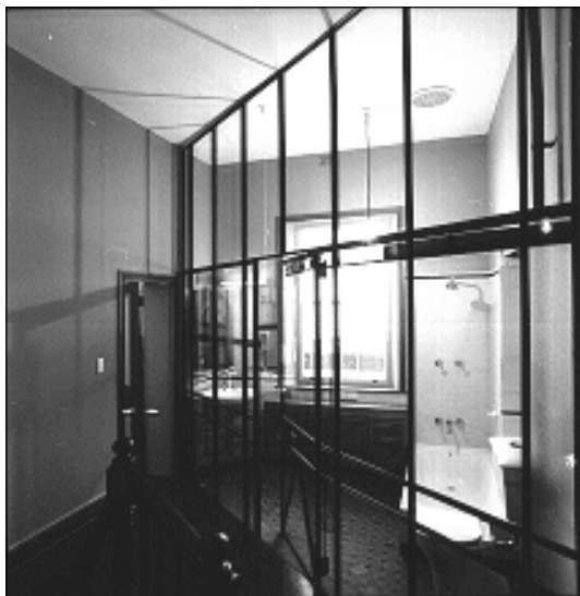
Figure 11: New bathroom facilities which allow the original space and character of the room to be appreciated
