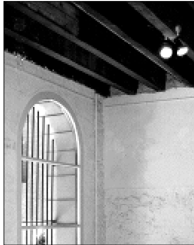
Figure 19: The side walls after repair
