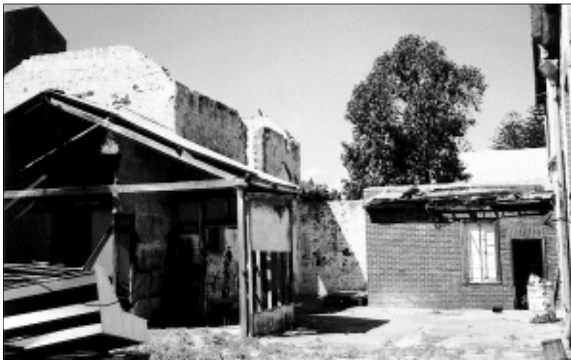
Figure 3: The former derelict rear Warehouse and Workshop
