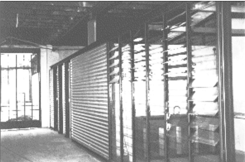
Figure 9: A new wall for the modern facilities constructed on the same plan as a former office wall in the Cartway.
