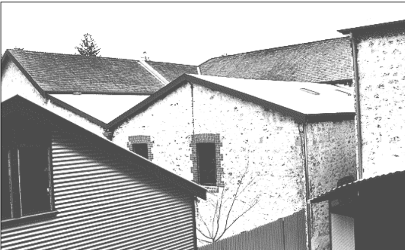
Figure 17: The former Warehouse roof was renovated using materials indicated by the evidence
