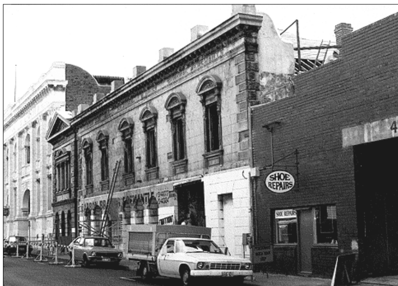
Figure 1: The Moores Building facade in 1986
