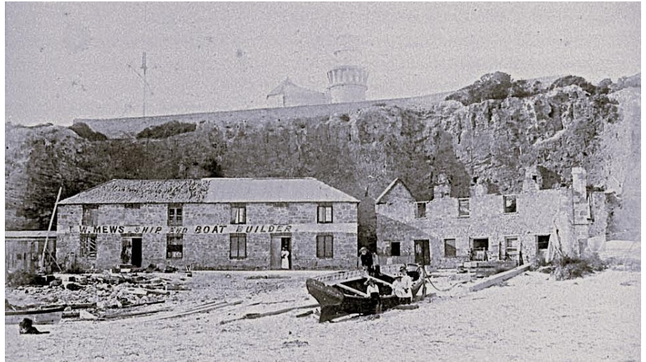
The bluff of Arthur Head, c. 1891. Fremantle History Centre (FHC) LH001614 On the right are the abandoned premises of the Fremantle Whaling Company
