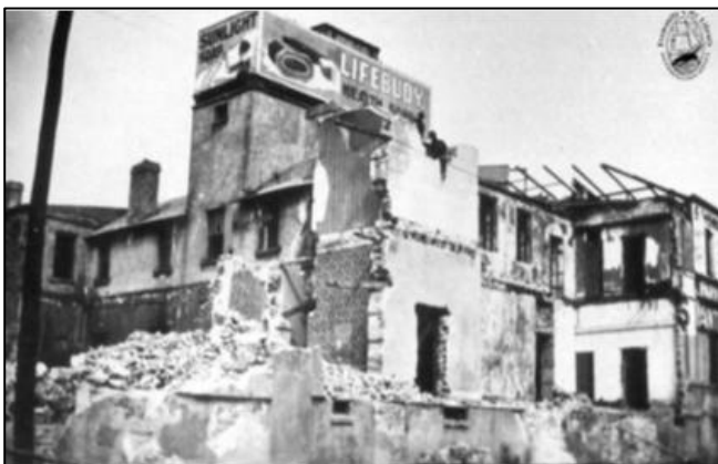
Demolition of 'Manning's Folly' 1928. FHC LH2048A
