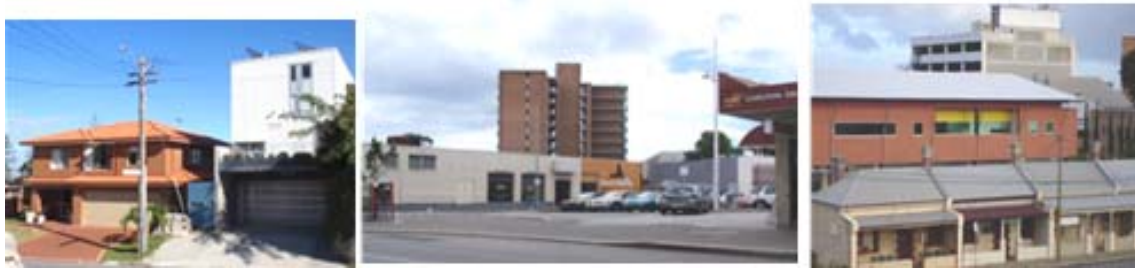
Figures 9, 10 and 11: Examples of infill developments representing an excessive margin of deformation according to the Code
