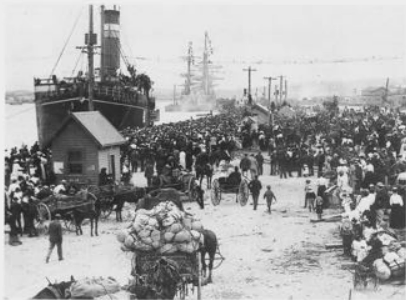
South Quay (later Victoria Quay) had to handle major crowds with primitive facilities in its early years as the Daily News and others complained. Here, in one of the most evocative and telling photographs of the port's 100 year history, is the Bushmen's Contingent setting off to the Boer War in March 1900 aboard the "Maplemore." A.O. Neville, who had so much to do with immigration and tourism through Fremantle, helped organise the contingents for the Boer War, one of which included his brother Frederick. (WAN Hist 5815)
