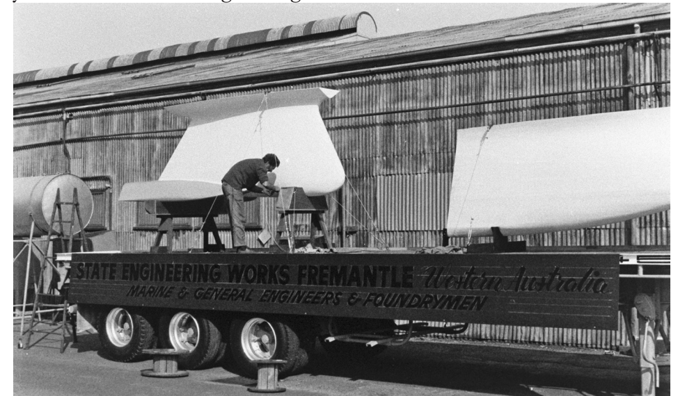
Image 5: The pattern for the keel for Australia II was made in the Eastern States and the keel was cast in the new foundry at the State Engineering Works, 1983. Image Credit: City of Fremantle History Centre [LH004002]
